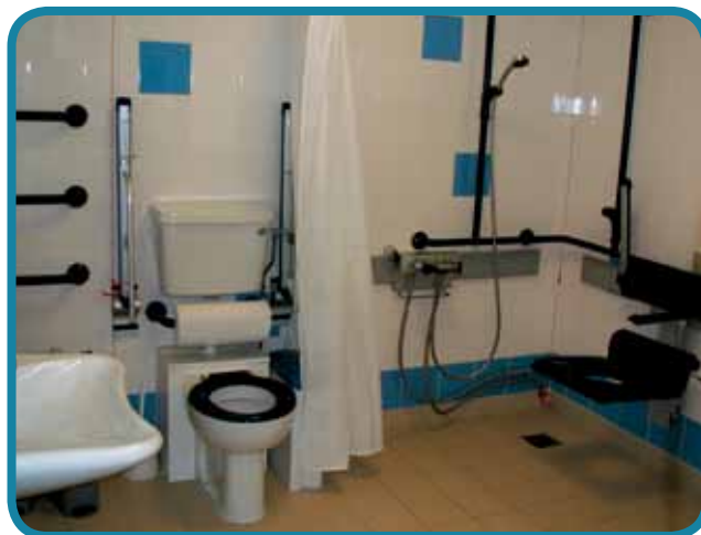
The CP facility at Ken Martin Leisure Centre in Nottingham includes a shower seat with a backrest and drop-down arm supports
